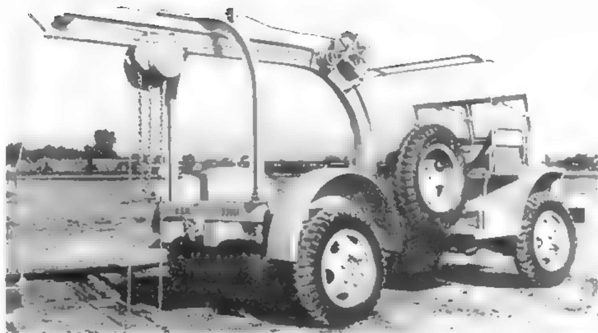
The GTBS was the first variant used by the Navy for a bomb service truck. In this photo the single rear tires characteristic of the GTBS are visible. This truck lacks a front winch. (Photo courtesy of the Bryce Sunderlin collection)
